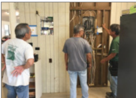
In late February, the B&G team did the project of rewiring Kanda Hall and adding a more robust electrical breaker panel for future expansion of circuit breakers and electrical loads—specifically, in anticipation of installing the new 220V AC unit that was donated to the church by an anonymous donor last Christmas. Although they had to hire an electrician contractor—Jeff Takemoto—B&G was able to do this project inexpensively by doing some of the rewiring work themselves (Dennis and Daniel spent hours crawling and working in the cramped space underneath Kanda Hall—see photo on the right.)
