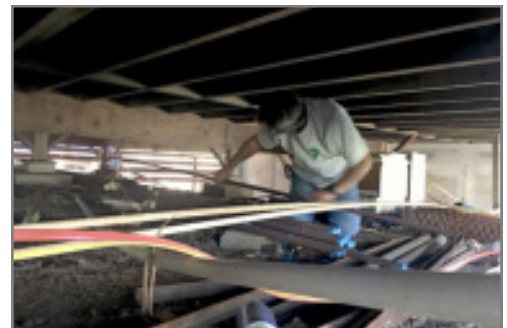
In late February, the B&G team did the project of rewiring Kanda Hall and adding a more robust electrical breaker panel for future expansion of circuit breakers and electrical loads—specifically, in anticipation of installing the new 220V AC unit that was donated to the church by an anonymous donor last Christmas. Although they had to hire an electrician contractor—Jeff Takemoto—B&G was able to do this project inexpensively by doing some of the rewiring work themselves (Dennis and Daniel spent hours crawling and working in the cramped space underneath Kanda Hall—see photo on the right.)
